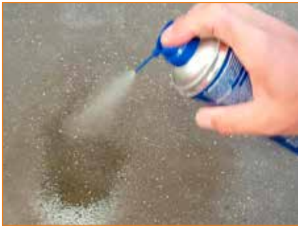
Degrease the surface.
